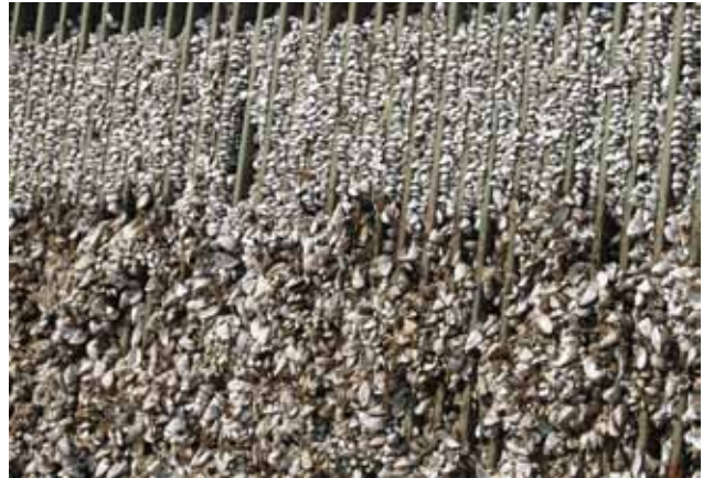
The zebra mussel can cause damage by blocking pipes, vents and any holes or openings where water flows. Reservoir tower safety grating clogged with zebra mussels (Rabisha Reservoir, Bulgaria).
