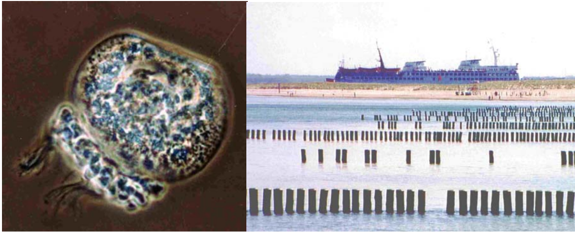
Fig 3. Shipworms veliger larva with characteristic ring of cilia. Fig. 4. Shipworm induced losses of groyne field piles built to protect sandy coasts from erosion cause substantial economic harm in Mecklenburg-Western Pomerania region of Germany. Photos by Dr. Jenz Gercken, Institute for Applied Ecology, Rostock.
